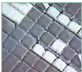
Loss of interlayer adhesion
